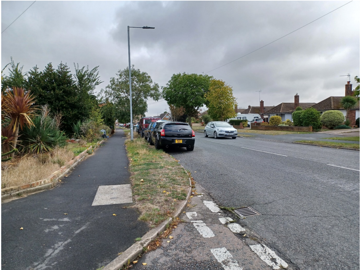
Sherwood Drive junction with London road – vehicles obscuring view from vehicles exiting.
